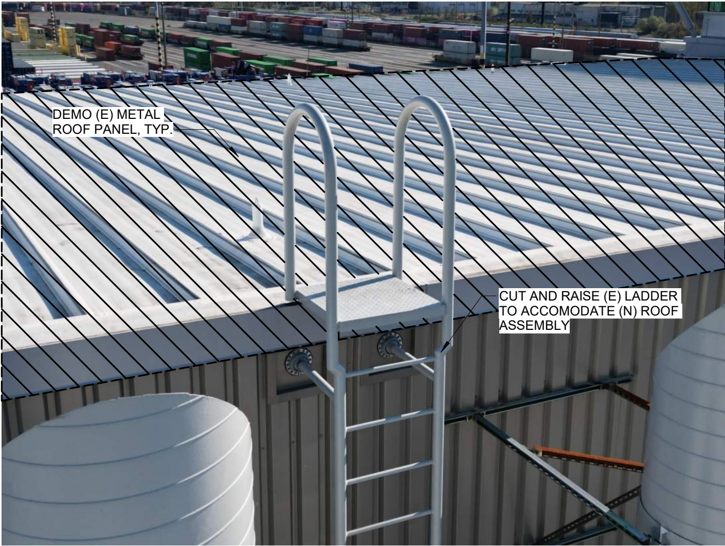
8 (E) ROOF ACCESS LADDER AD9.10 NTS
